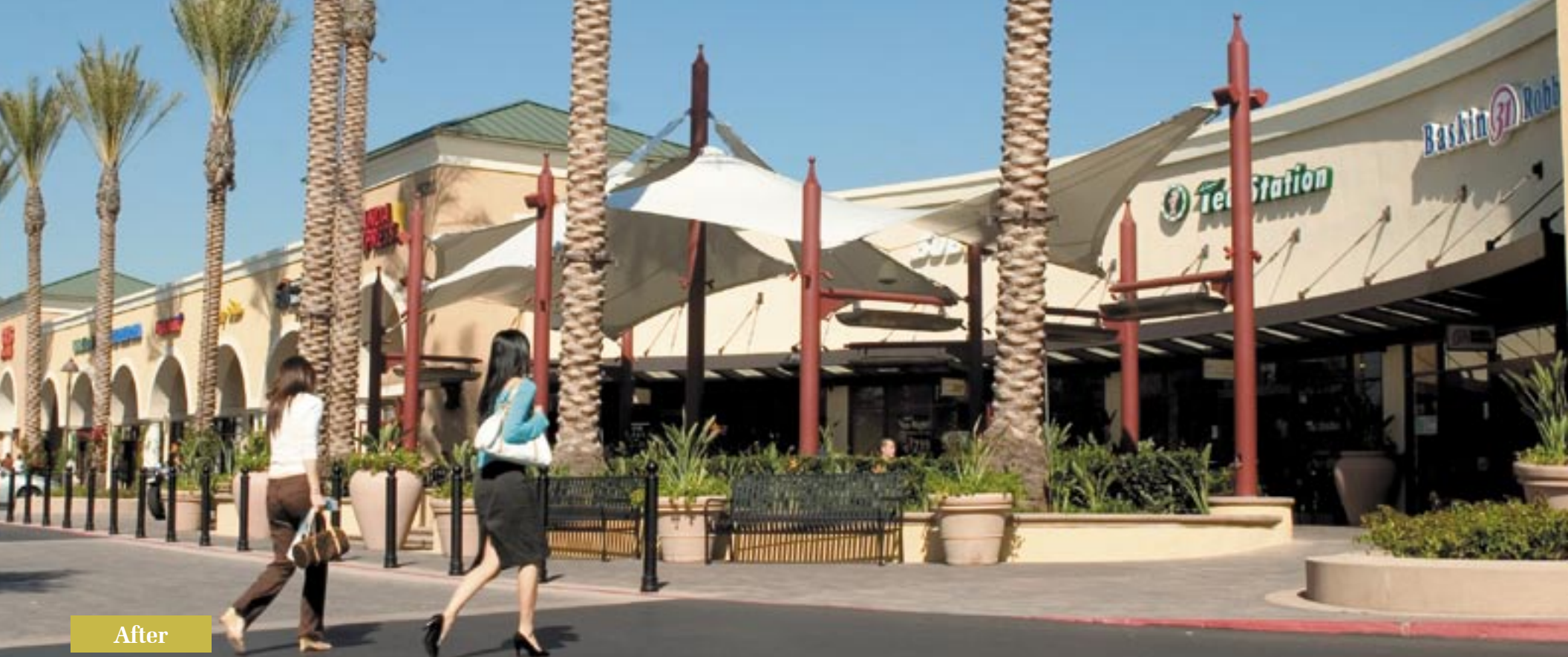
Culver Plaza after its renovation.
